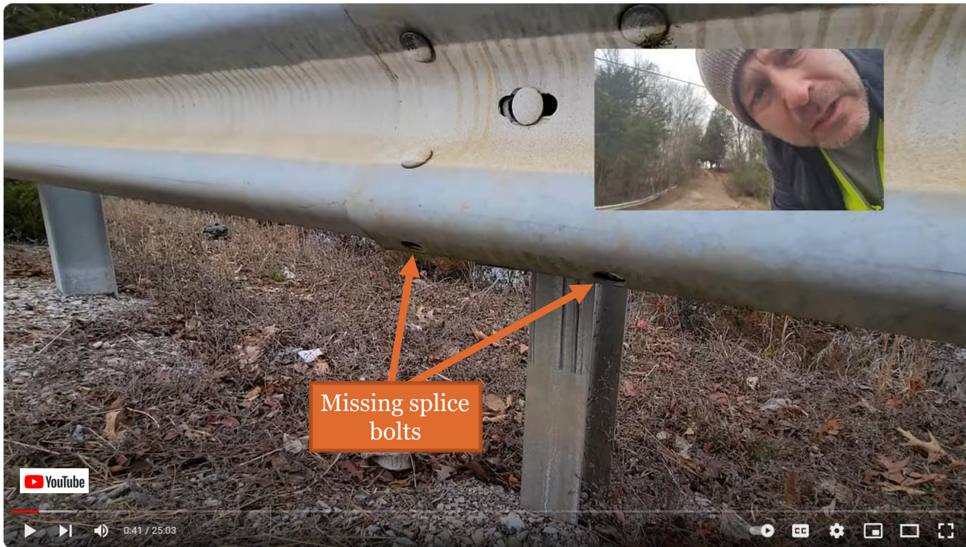
Lake Guardrail MISSING over 200 Splice Bolts
