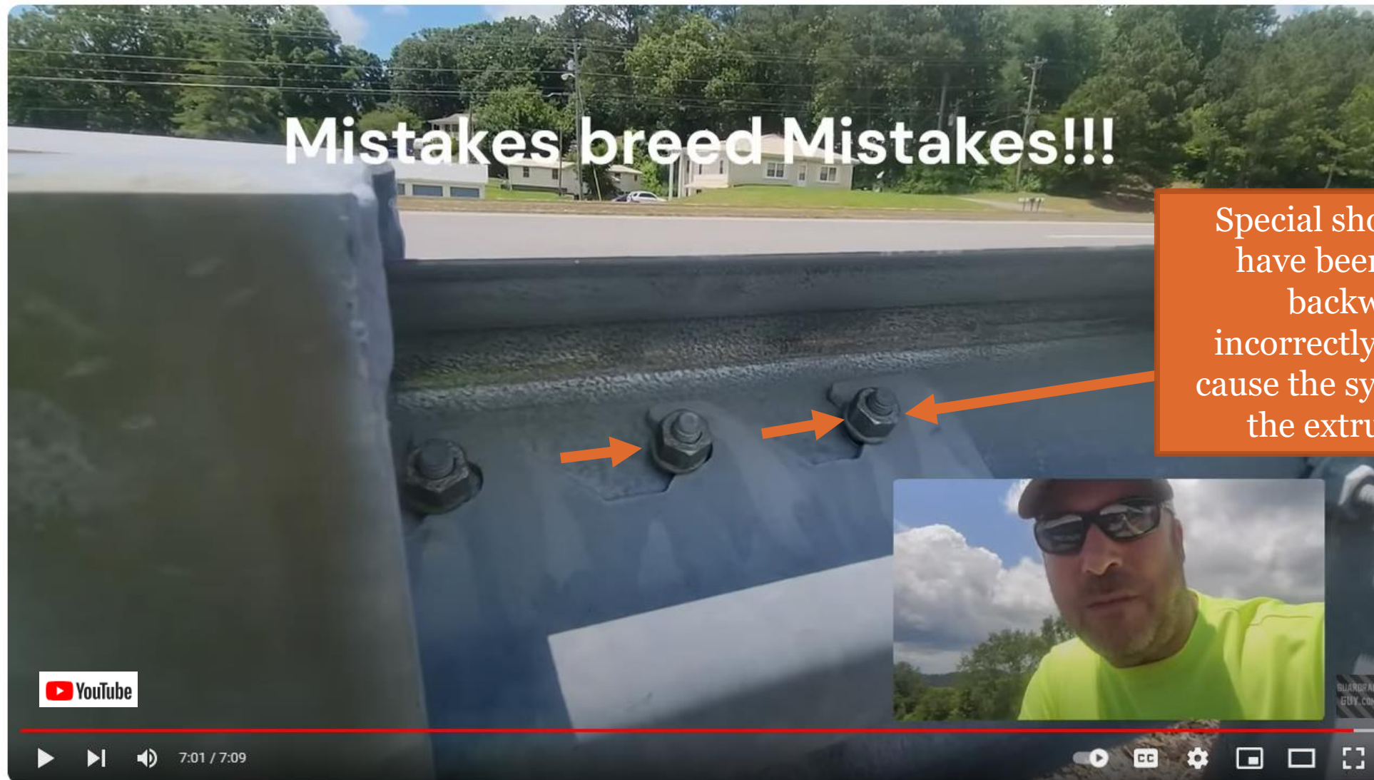
Explanation of Backward Bolts Guardrail Short with Million+ Views
